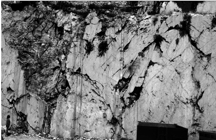
Fig. 10. A sawn face 10 m high on a construction site sections limestone just below rockhead in a karst of class kIV in northwestern Sicily. Small caves and dissolutional-opened fissures are mainly aligned on dipping fractures, and a buried sinkhole is exposed on the left after its fill has been removed. Note person at lower left of image for scale.
