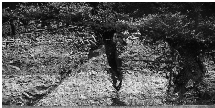
Fig. 11. A road cutting 4 m high in class kII karst in Korea, exposing two clay-filled sinkholes cut below a rockhead with minimal fissuring.
