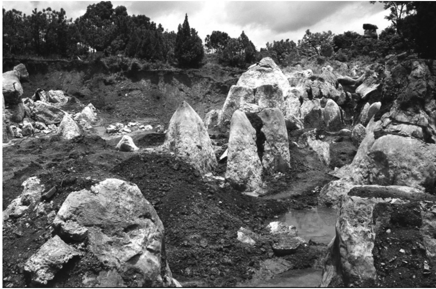
Fig. 8. Pinnaced rockhead partially exposed on a construction site in class kV ground at Lunan, in Yunnan, China. The original ground surface had only a few protruding pinnacle tips. Excavation to a lower level achieves a greater proportion of rock to soil for bearing purposes, but requires removal of the taller pinnacles.
